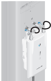
Connecting to a Sector Antenna
