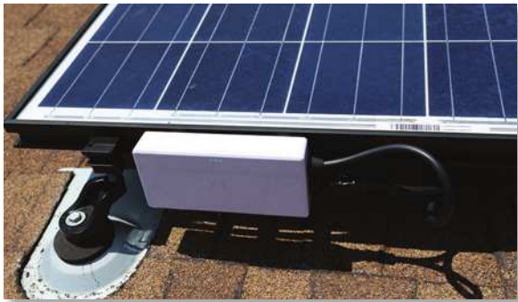
Solar Gateway Installed
