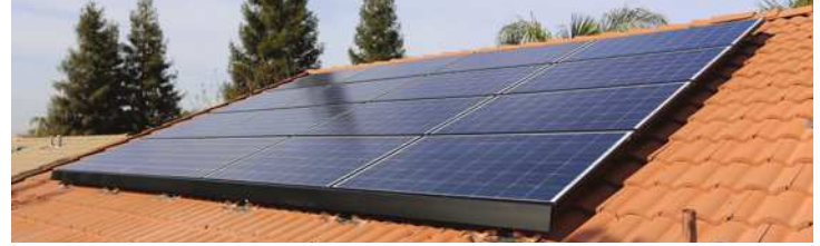
Four Landscape Trim Covers Installed
